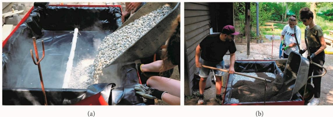
**Figure 13.** Construction work on the filter trough. (a) The drainage layer consists of 15 cm of gravel. (b) A layer of lava sand follows the gravel.
